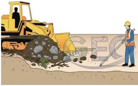
1. Prepare subgrade. Remove debris, rocks.
