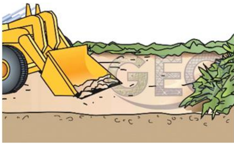
1. Prepare subgrade. Remove debris, rocks.
